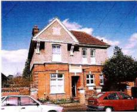
Edward House, 79 Southampton Rd, Fareham (2 flats for couples)
