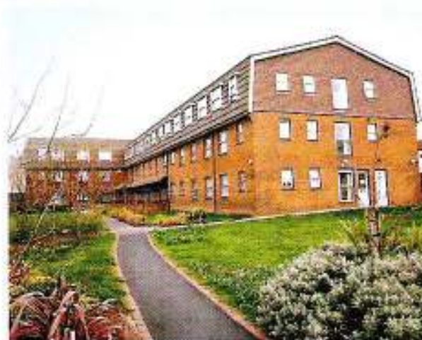
Harrison House, Stamshaw Rd, Portsmouth (28 1 bed flats, 2 double flats)
